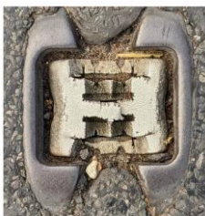
Most of the road studs (x102) are in this condition
