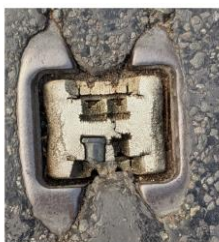
Example of road stud with 1 remaining cat's eye (compacted below road surface)
