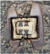
Only remaining road stud (this 70) with 3 cat's eyes compacted below road surface
