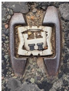
Only remaining road stud (No. 77) with 2 cat's eyes (compacted below road surface)
